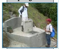
Spring water is usually drinkable as it comes from the ground but it can get contaminated by animals and other sources as it collects at the spring head. A spring box collects the water and protects it from contamination. The clean water is then piped to water stations below the spring in the communities where the water is needed.
