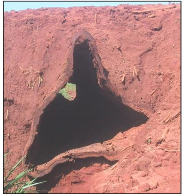
One way to make a culvert!
