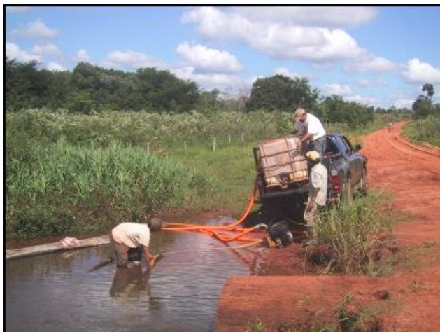
We have a new way of getting water to the job site, much easier and faster
