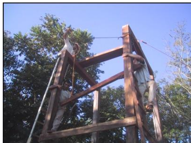
Guys building tower – all done by hand & ropes
