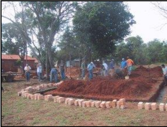
Building the foundation
