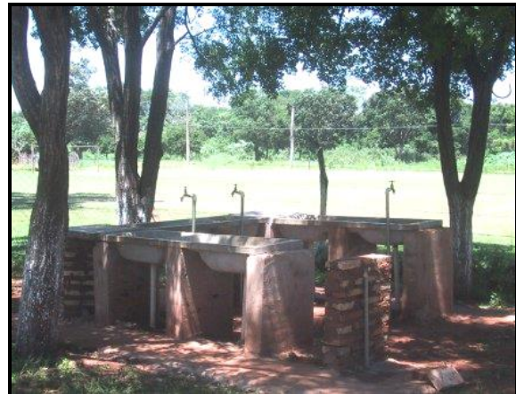
New 3 sink wash station, no more taking laundry to the creek!
