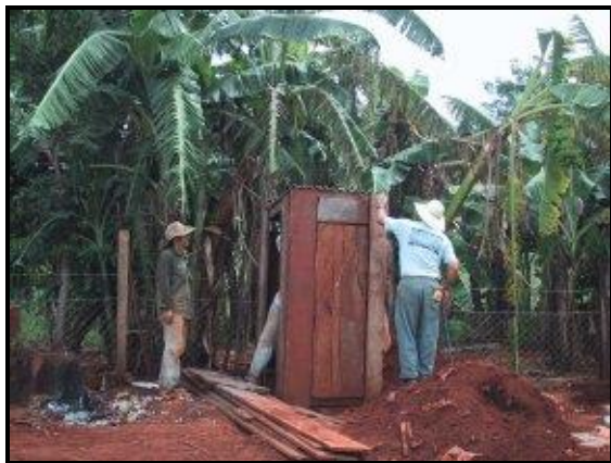
Tearing down old outhouse – Adios!
