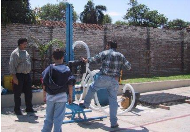
Starting rig for the 1 st time
