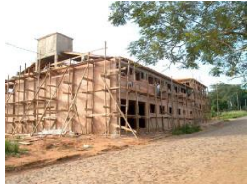
Methodist school under construction
