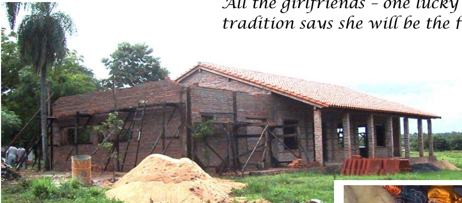
Kitchen addition to the Multi-Use facility
